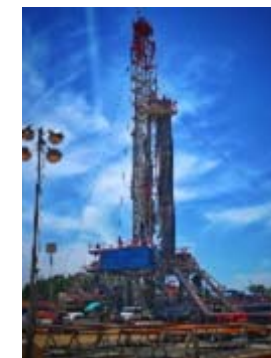
Sabine Oil & Gas Corporation (Shale gas well drilling site)
