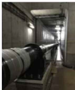
Amagasaki–Kumiyama Line (Construction status)
