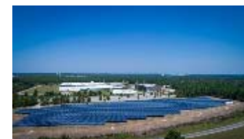
Solar power plant in USA (SolAmerica Energy, LLC)
