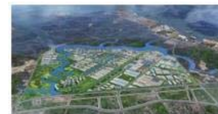
City gas supply in Phu My 3 Specialized Industrial Park in Vietnam
