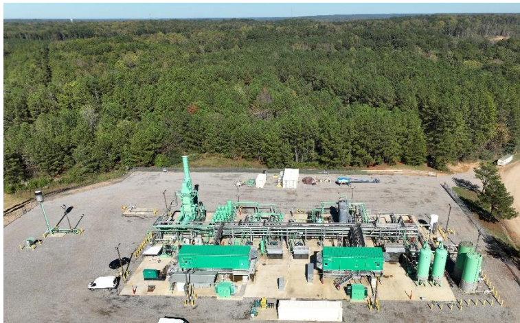
View of a landfill-based biomethane production facility (Courtesy of Archaea Energy)
