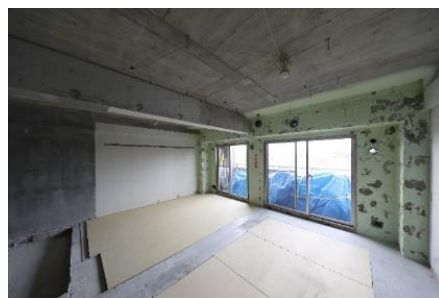
② After dismantling
