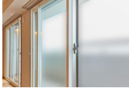
⑤ Interior window (Low-E double-glazed glass)
