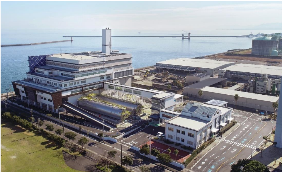
Photo: Exterior of the Kagoshima City Nanbu Incineration Processing Plant (courtesy of Kagoshima Municipal Government)
