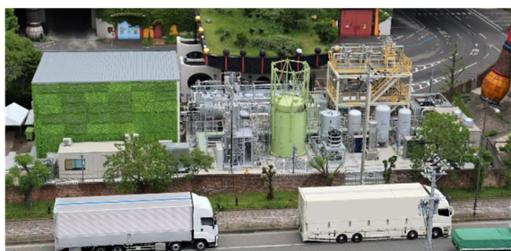
Exterior of the methanation demonstration facility
