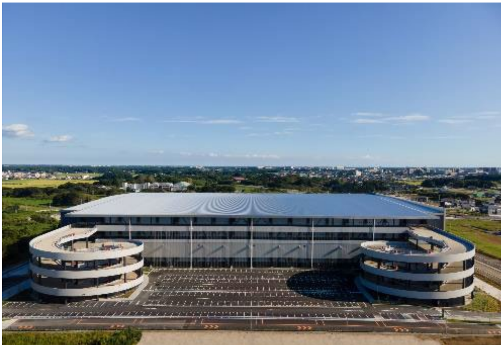
(Tsukuba City, Ibaraki Prefecture/Installed capacity: approx. 3,500 kW)
