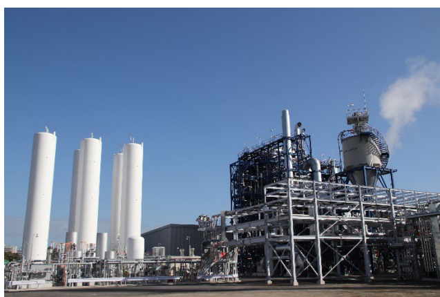
Exterior view of the new thermal power plant
