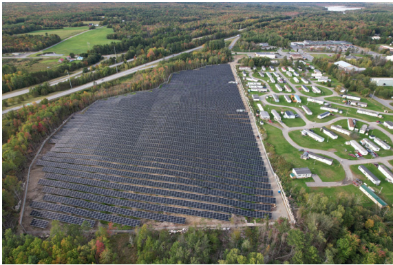
Fig. 3 CS project in Maine with SRE
