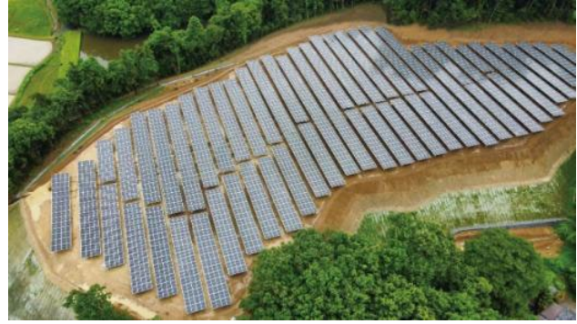
Solar power plant in Yamada, Namegawa Town, Saitama Prefecture (Installed capacity: 1,870 kW)
