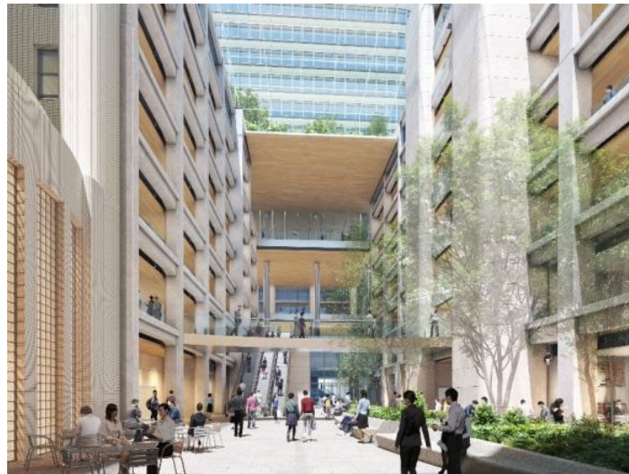
Image of the Gas Building atrium
