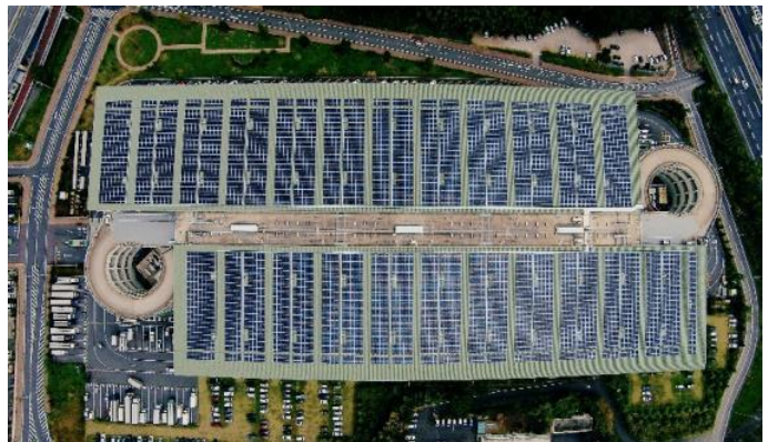
Power plant viewed from directly above
