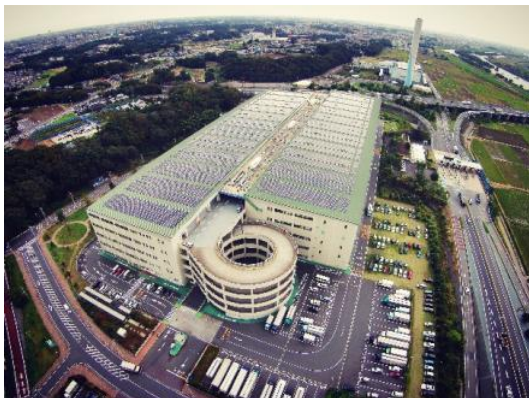
Solar power plant on rooftop
