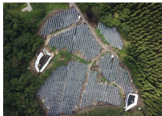
Shinano-machi Solar Power Plant
