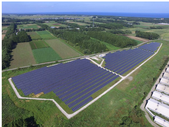
Misawa Solar Power Plant
