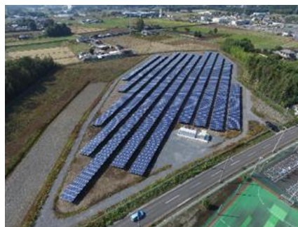
Haru Mito Solar Power Plant
