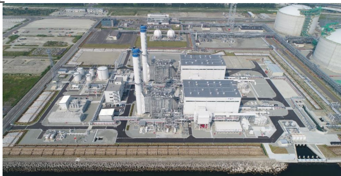
Overall view of the power plant
