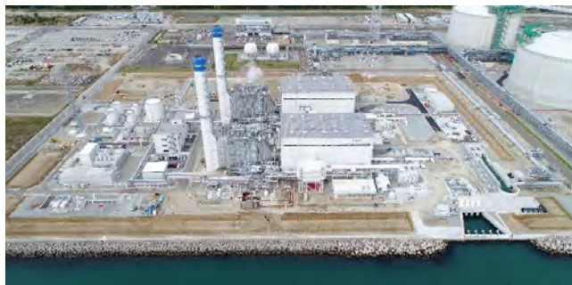
Overall view of the power plant
