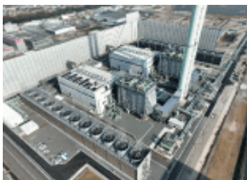
Himeji Natural Gas Power Plant (Hyogo Prefecture)
