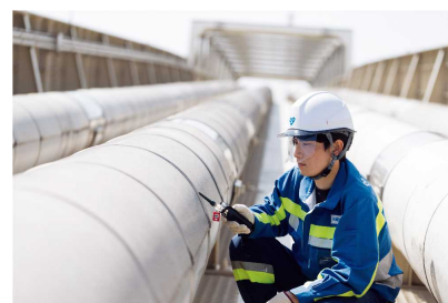
Bridge pipe safety inspection
