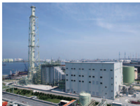
The Senboku Natural Gas Power Plant
