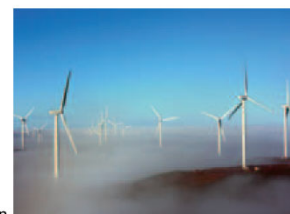
"Hallett 2" which is operating near "Hallett 4" under construction
