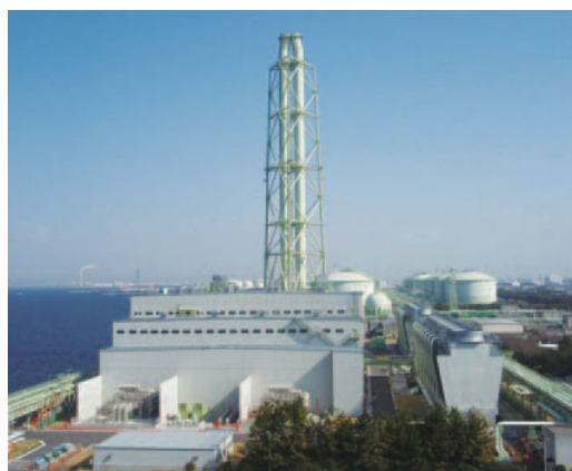
The Senboku Natural Gas Power Plant
