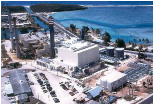
The Marianas power plant in Guam,US
