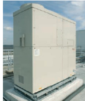
The “GENE-LIGHT” gas engine which enables use of exhaust heat for cooling
