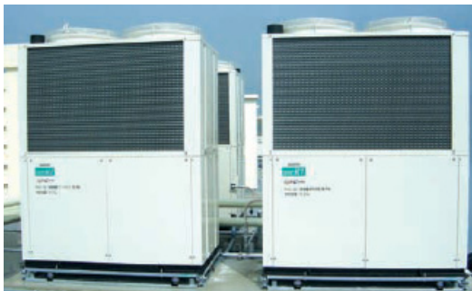
The “HIGH POWER EXCEL” gas heat pump-type air conditioning system with functions for electric generation and air conditioning
