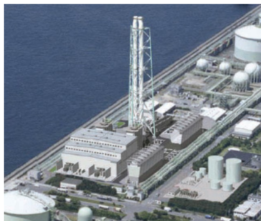
Completion image of The Senboku Natural Gas Power Plant
