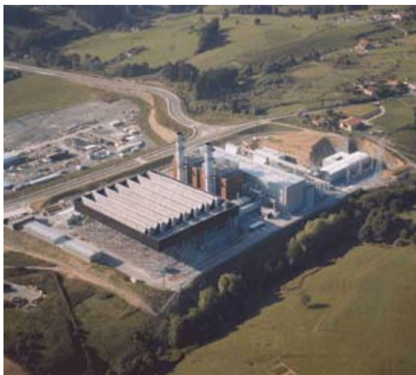
Amorebieta power plant
