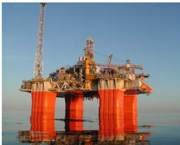
marine drilling platform in the North Sea oil field (photo by Idemitsu Snorre Oil Development Co., Ltd.)
