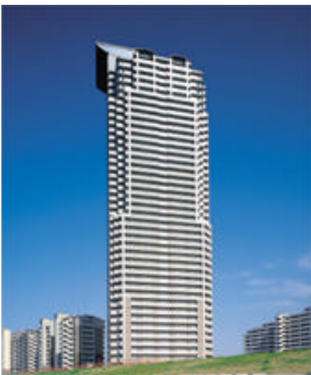
Complex housing employing the gas cogeneration system
