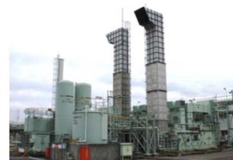
Enhancement of backup power generation facilities at terminals by replacing oil power generators with gas types
