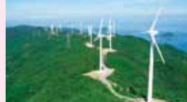
Wind Power Generation Business
