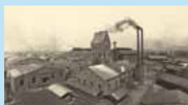
Foundation / commenced gas operations
