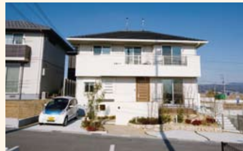
House used as an experimental dwelling (Kitakatsuragi District, Nara Prefecture)
