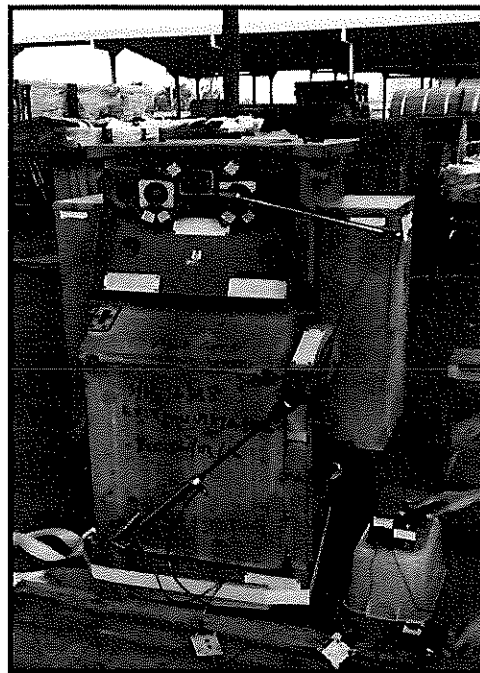
Figure 1: The attachment of a safety switching system to the switchgear.
