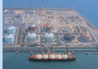
Himeji LNG Terminal at start of operations (Hyogo Prefecture)
