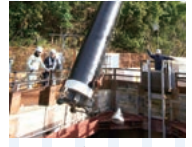
Himeji-Okayama Gas Pipeline construction
