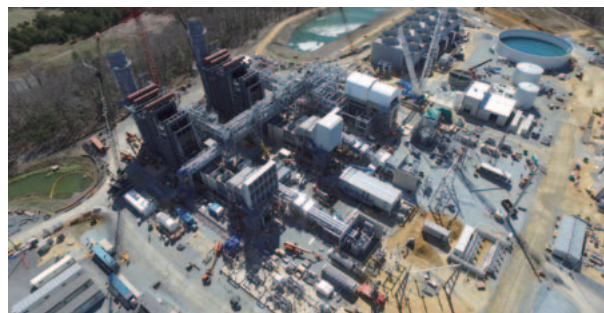
St. Charles Energy Center Natural Gas-Fired Power Plant (under construction)
