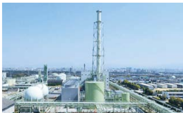
Semboku Natural Gas Power Plant (Osaka)
