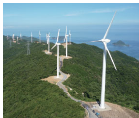
Hirogawa Myojinyama Wind Power Plant
