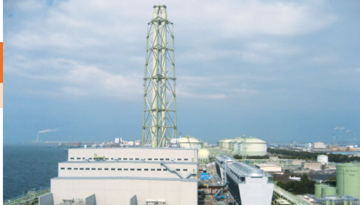
Semboku Natural Gas Power Plant
