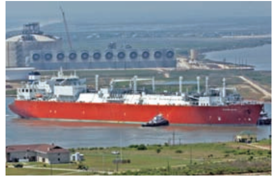
LNG receiving terminal in Freeport, Texas in the U.S. (Photo courtesy of Freeport LNG Development, L.P.)
