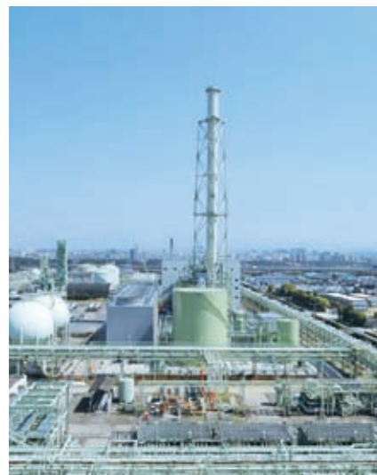
The Semboku Natural Gas Power Plant
