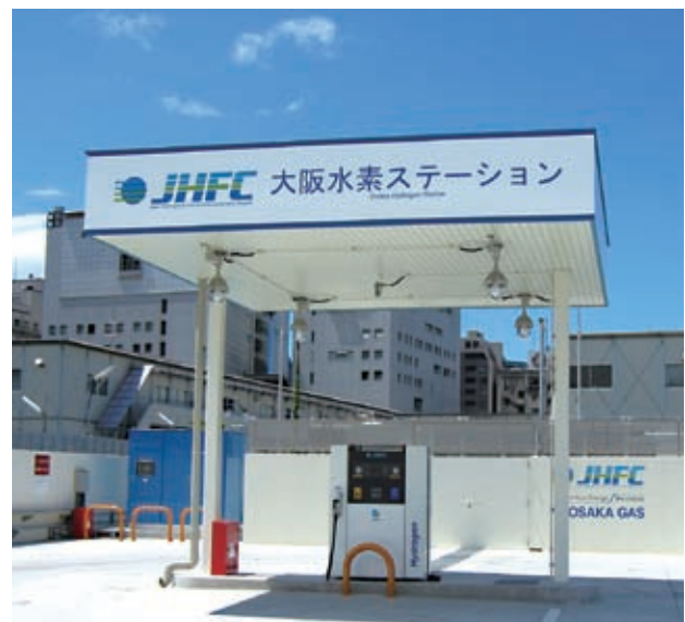
Japan's first urban hydrogen supply station (Osaka City)
