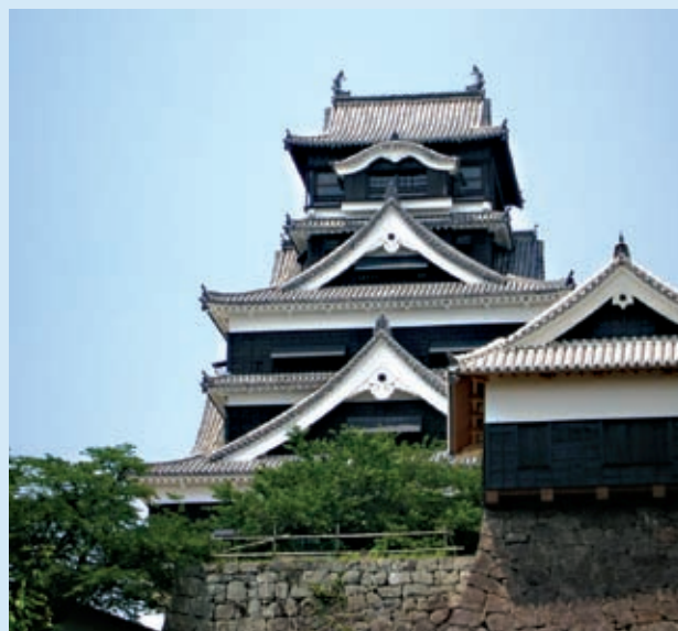
Xyladecor, a decorative wood preserving stain produced by Japan EnviroChemicals Ltd., is used at a number of Japanese National Treasures and Important Cultural Properties (Photo: Kumamoto Castle)
