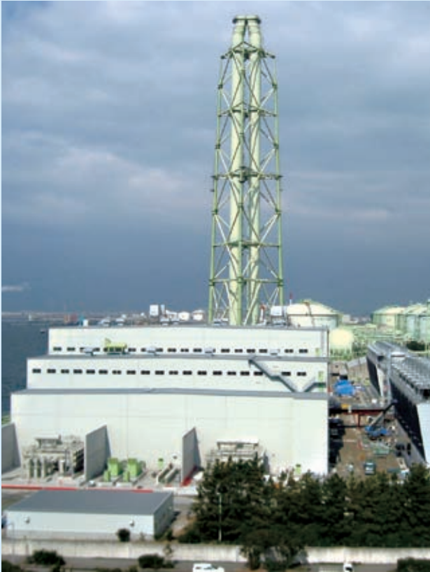
The Semboku Natural Gas Power Plant, scheduled for completion in 2009
