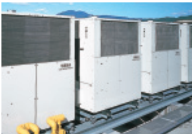
A commercial-use High Power Excel GHP unit with a generator function to supply power while it is providing air conditioning
