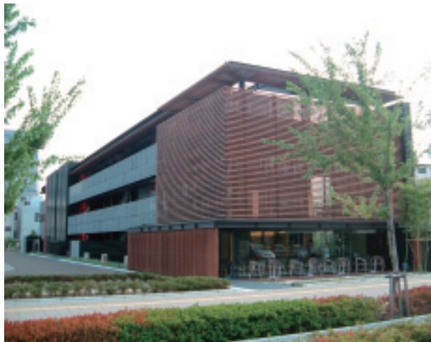
The newly completed No.8 Building of the Kyoto Research Park, a new industry creation base in Kyoto.
