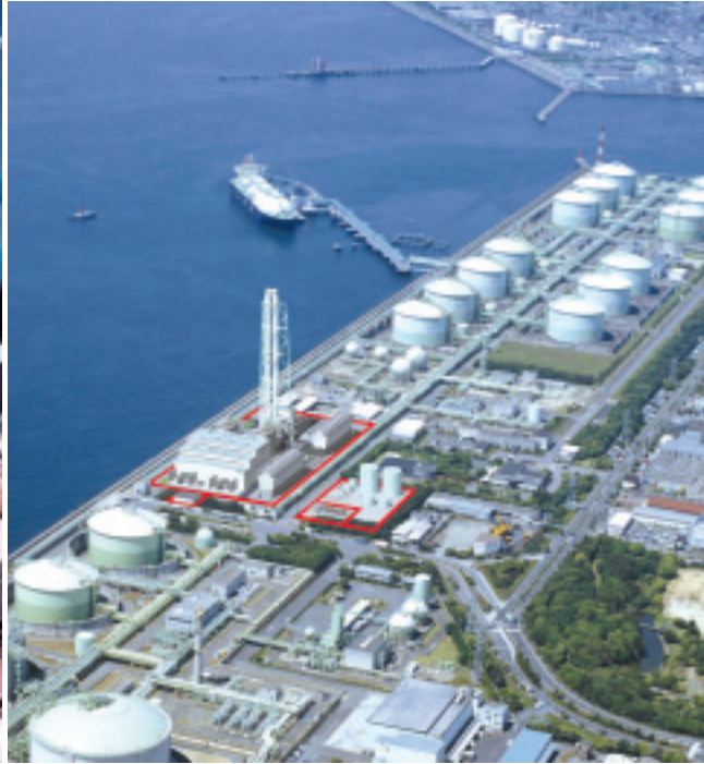
Rendering of the Semboku Natural Gas Power Plant.
