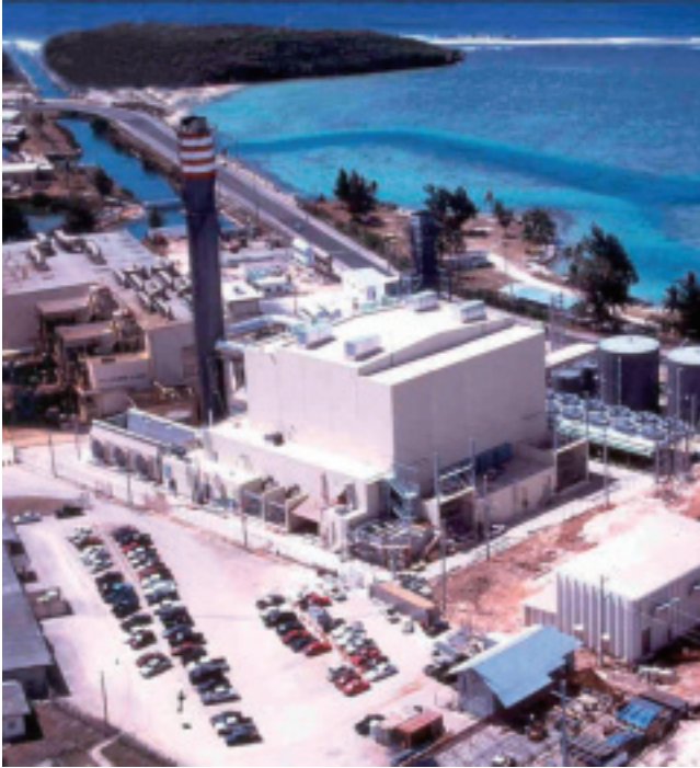
The Marianas Power Plant in Guam, for which the Osaka Gas Group owns 100% of the interest.
