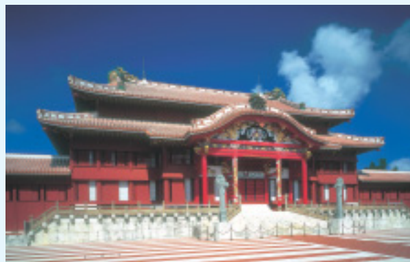
The wood structures of Shuri Castle in Okinawa Prefecture are coated with high-performance wood preservative manufactured by Japan EnviroChemicals, Ltd.
