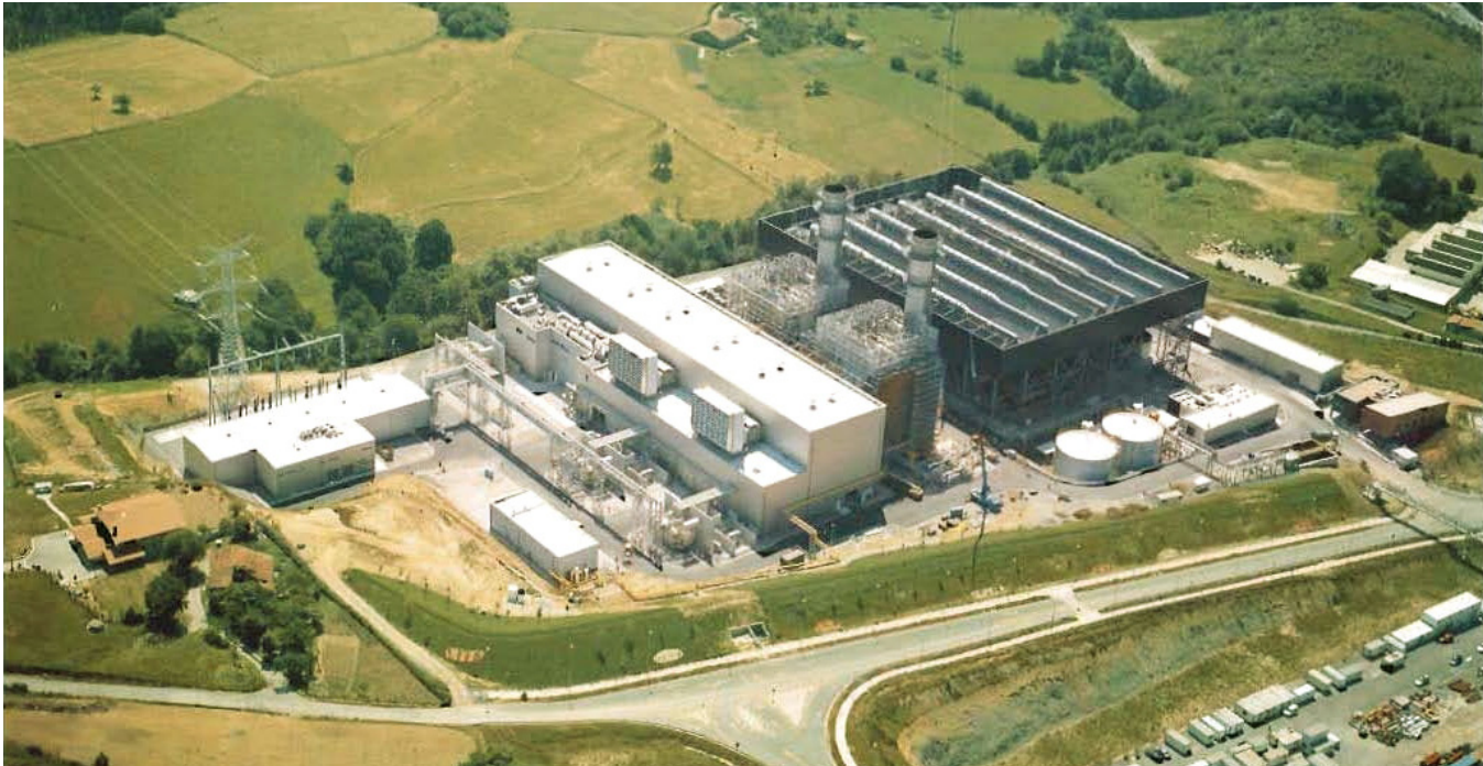
IPP facilities in Spain Osaka Gas financed in 2005
