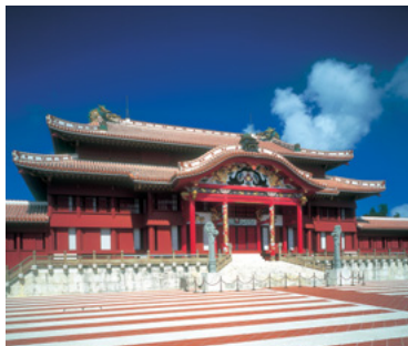
Shuri Castle in Okinawa Prefecture using high-performance wood protective coating from Japan EnviroChemicals
