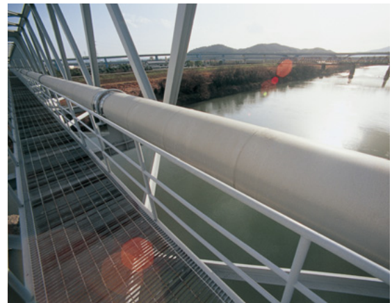
Ujigawa Pipeline Bridge
