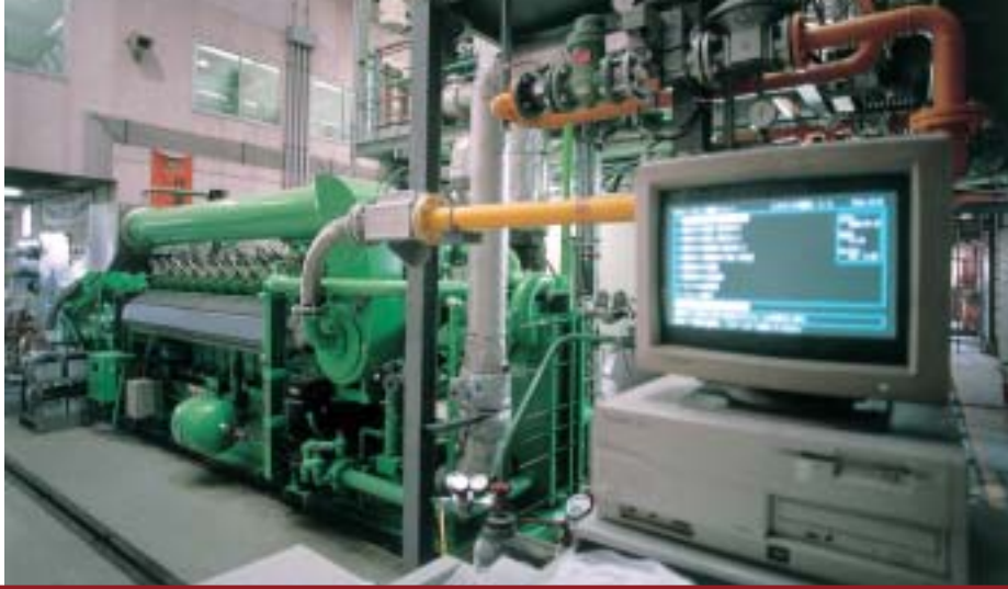
Featuring cutting-edge technology, this 1,000kW-class high-efficiency engine boasts power generation efficiency of approximately 41%.
