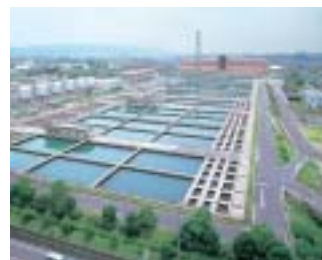
Using waste heat from cogeneration in the cleansing process at a water purification plant
