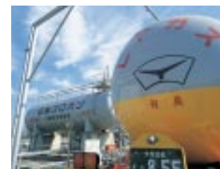
An LPG replenishing facility
