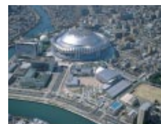
Iwasaki-Bashi Area District heating and cooling system
