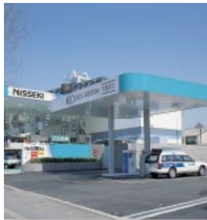
Eco-Station (Natural Gas Stand)
