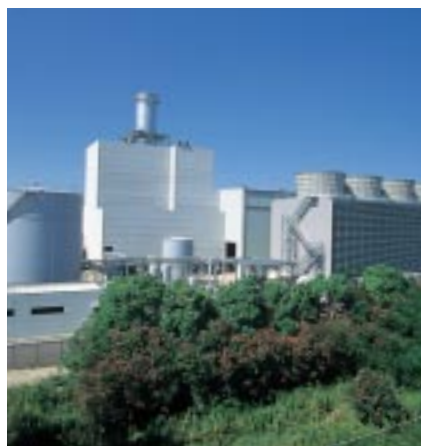
The Torishima Energy Center
