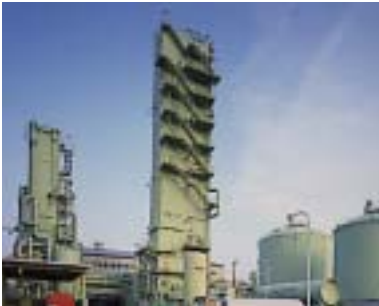
An air-separation plant of the Liquid Gas Group.
