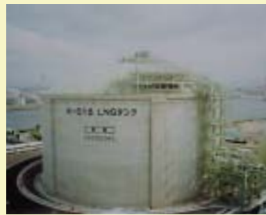
The No. 18 LNG tank at the Senboku Terminal.
